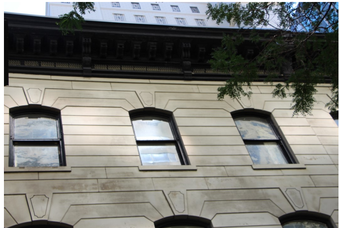
Window and door openings are arched and topped with projecting keystones. Horizontal joints in the limestone are exaggerated, and the row retains its original pressed-metal cornice, all features of the Italianate style of architecture.
