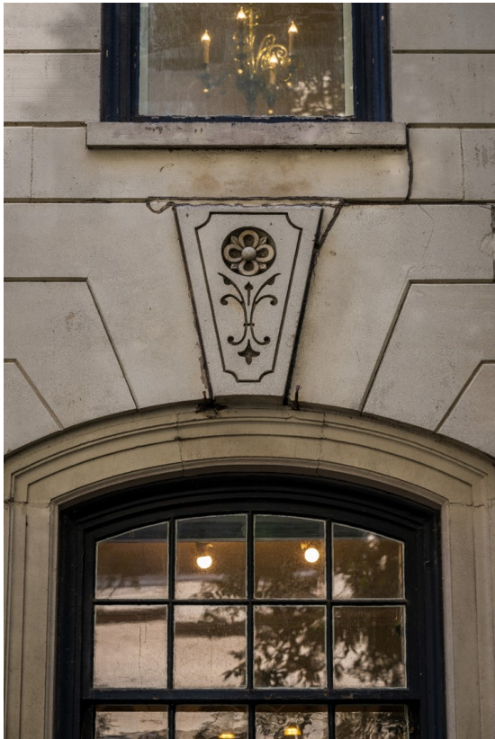
Window and door openings are arched and topped with projecting keystones. Horizontal joints in the limestone are exaggerated, and the row retains its original pressed-metal cornice, all features of the Italianate style of architecture.
