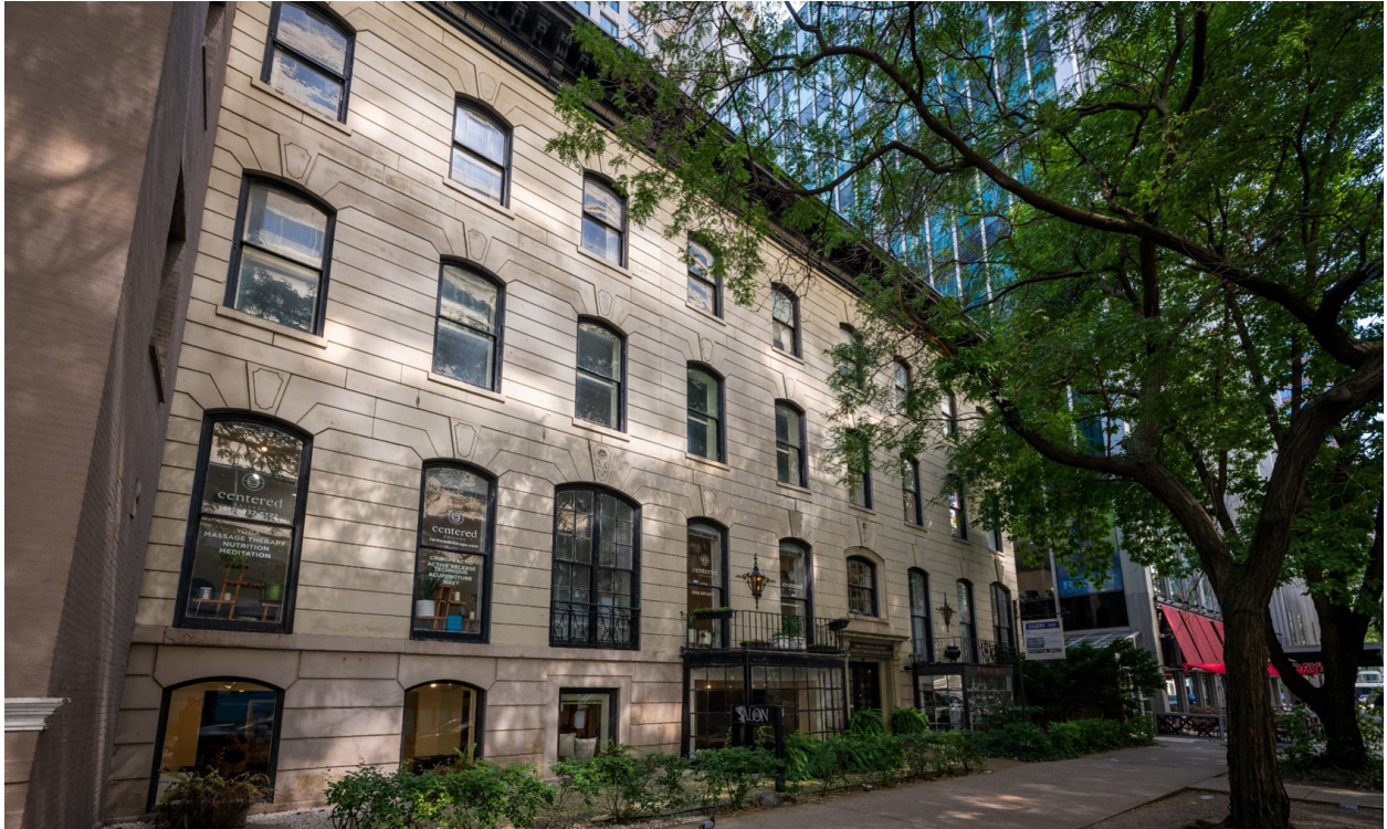
The Erie Street Row is a fine example of a very early party wall row house with a uniform design. Though painted, the front elevation is constructed of Joliet Limestone, Chicago's earliest building stone.
