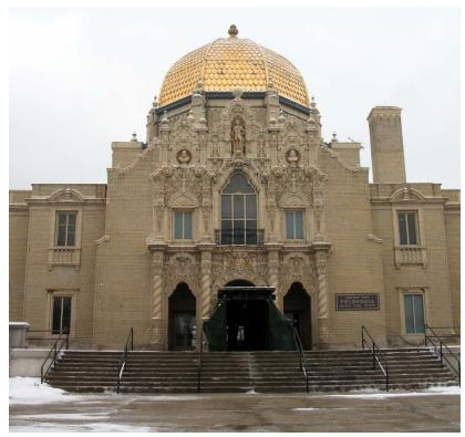
The central pavilion of the east elevation (above) with its exuberant "Churrigueresque" terra-cotta entrance portal and immense gold-leaf dome. The symmetrical wings on either side of the central pavilion are clad in cream-colored face brick laid in a distinctive Flemish bond.
