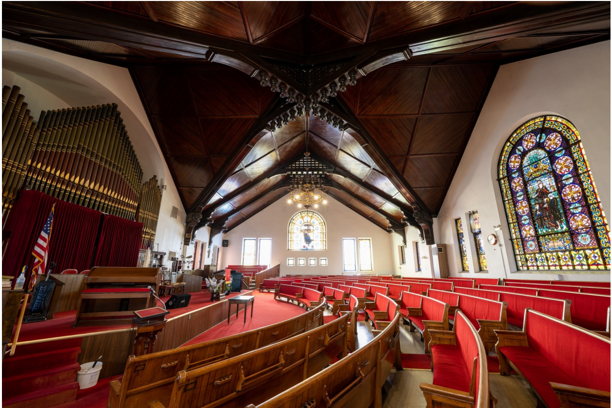
The capacious, bright and column-free interior of the worship space is supported by exposed hammer-beam trusses built up of laminated lumber. The ceiling is Southern pine with an oil finish.
