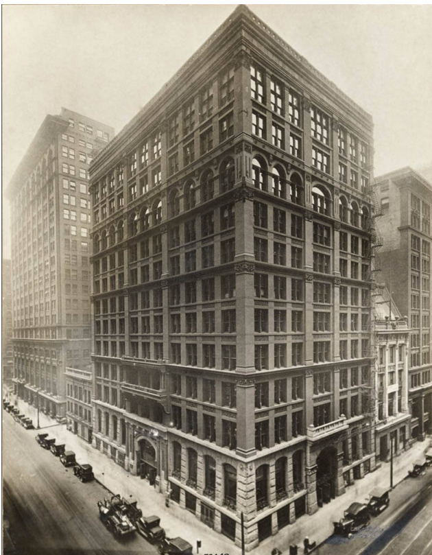
The Home Insurance Building at S. LaSalle and W. Adams Streets in Chicago is regarded as the world's first skyscraper due to its height and skeletal structural frame. It was completed in 1885 and demolished in 1931 to make way for the Field Building, a designated Chicago Landmark. (Credit: Ryerson & Burnham Archives Archival Image Collection)
