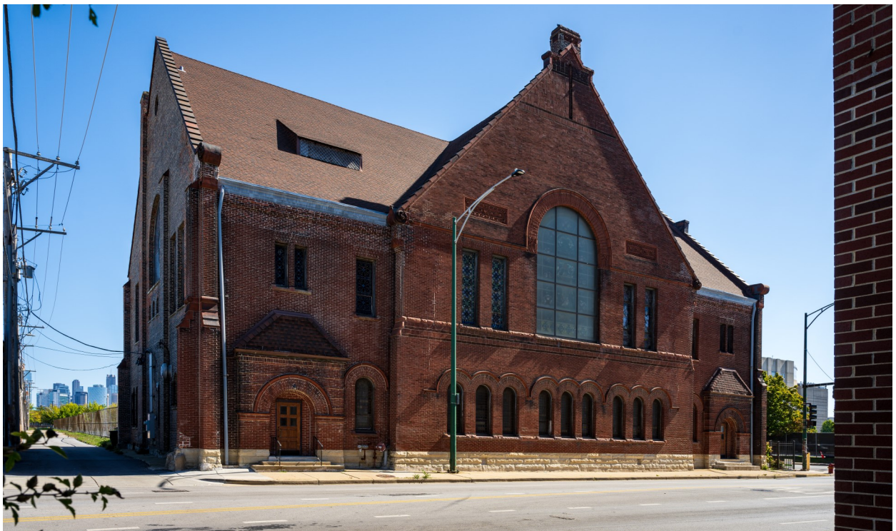
The west elevation facing Damen with an arcade of round-arched windows at the first floor and a cross-gabled roofline.
