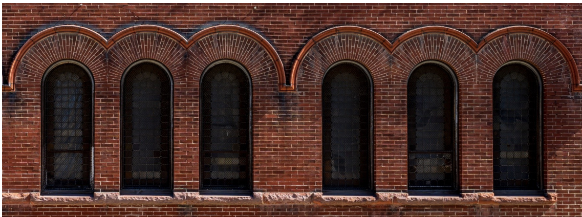
A selection of details from the building executed in unglazed terra cotta that are incorporated into the exterior wall structure.
