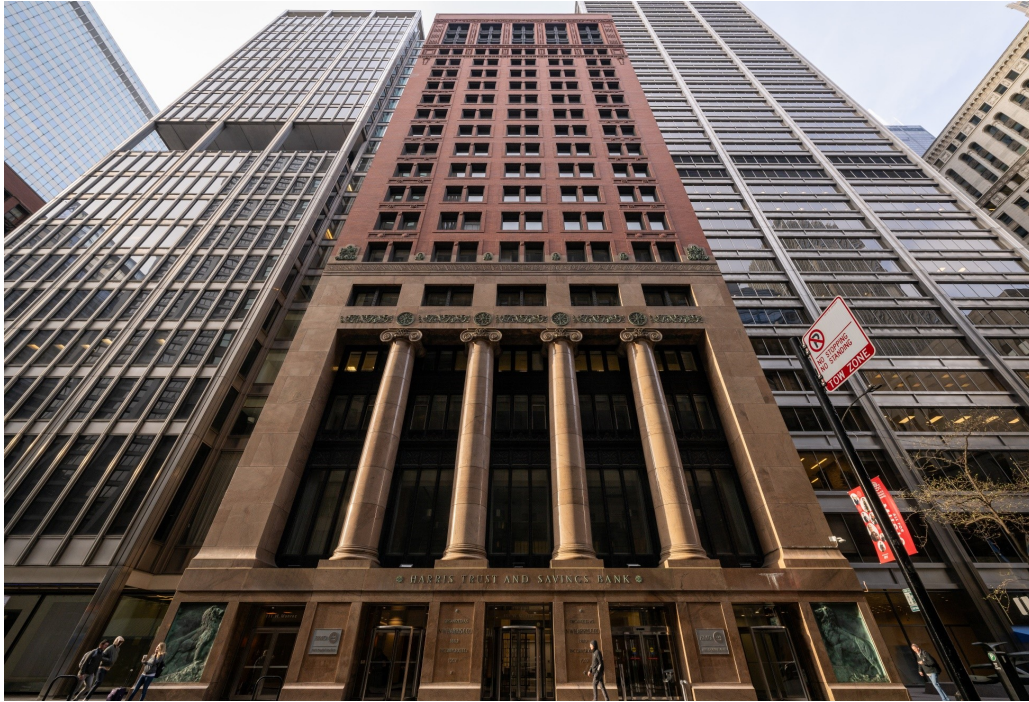
The building has a tripartite façade arrangement with a colonnade at its base, a smooth shaft in the middle, and more ornament at the top, though somewhat diminished by the loss of the original cornice.
