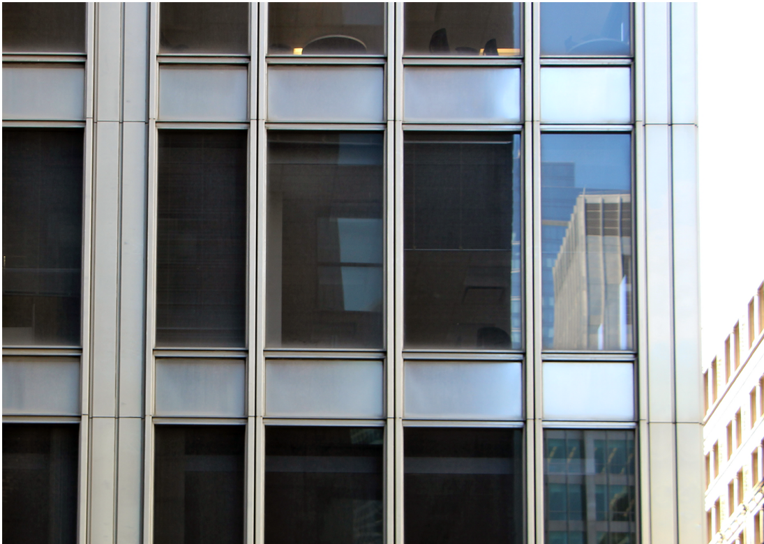
Details of the East Tower reveal an emphasis on brushed stainless steel detailing with precise design, fabrication, and installation.
