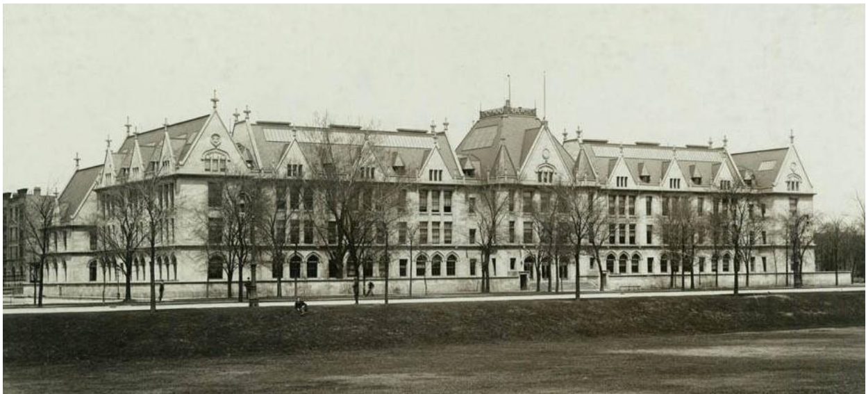
Above: Blaine Hall (1362 East 59th Street; extant) was built in 1903 for the University of Chicago's School of Education. Based on the Gothic Revival of Henry Ives Cobb's university buildings, its symmetry belies James Gambles Rogers's Beaux-Arts training. It is now the location of the University of Chicago's Laboratory School. (Source: Ryerson and Burnham Archives)
