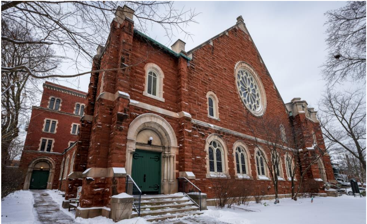
Below: Looking NW at the east elevation of Hyde Park Union Church. At left is the recessed portion of the building which gives a clear view of the Education Wing. (Photos by Patrick Pyszka)
