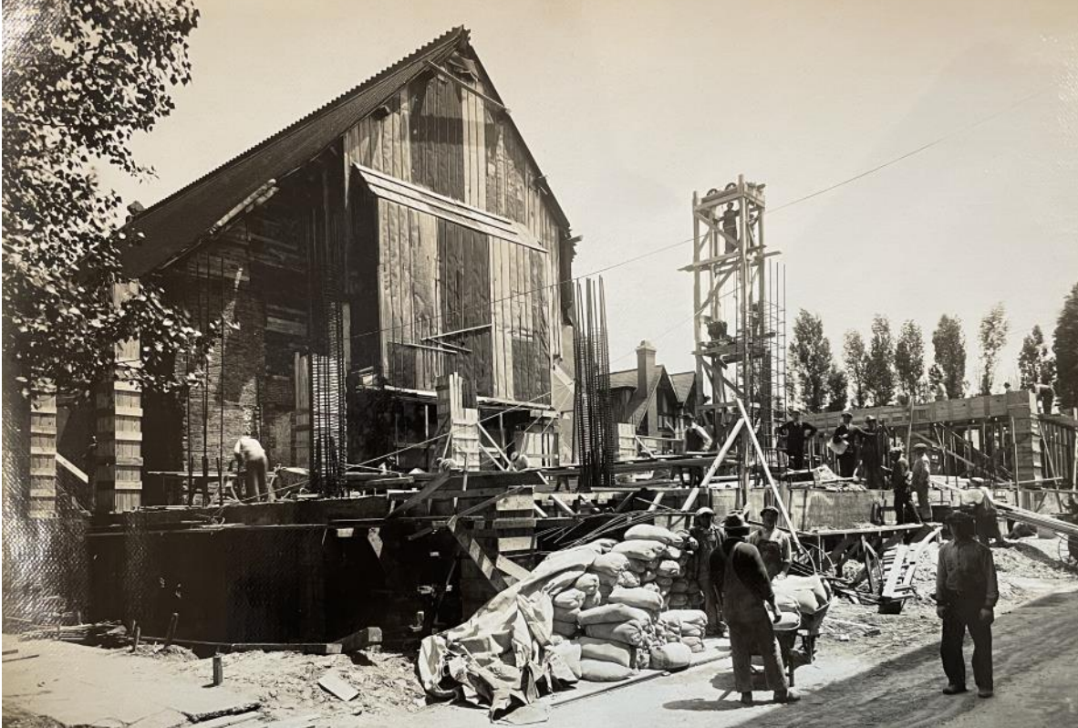
Above: During construction of the 1926 Education Wing addition, looking southeast. (Source: Hyde Park Union Church archives)
