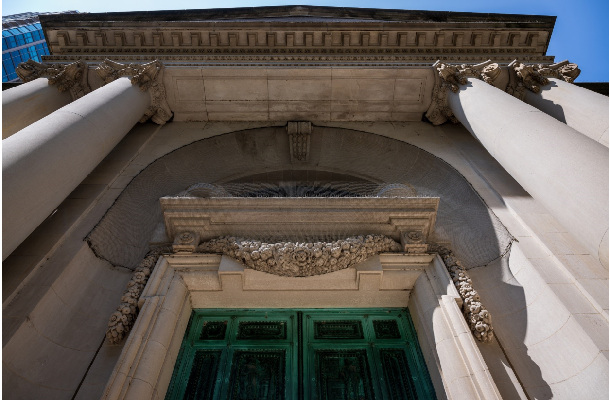
The building is abundantly detailed with high crafted cut limestone ornament. The building features a tall carved pediment (top), carved floral swags (bottom) are drawn from classical architectural traditions.
