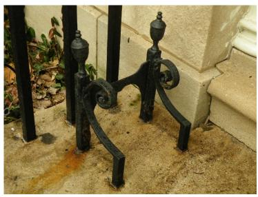
Image 25: Detail of wrought-iron boot scraper, each doorway features one on either side of the door.
