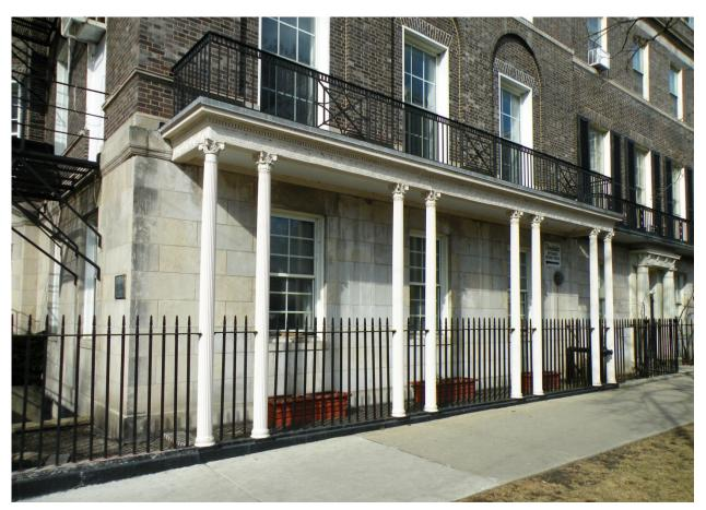
Image 40: Detail of cast-iron columns and balcony of number 2700.
