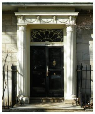
Image 8: 2704 North Lakeview Avenue. The main entryway for Abram Poole's house is flanked by fluted columns and has an entablature with a frieze featuring carved rams' heads and garland swags.
