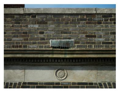
Image 23: Detail of limestone cornice and brick parapet.
