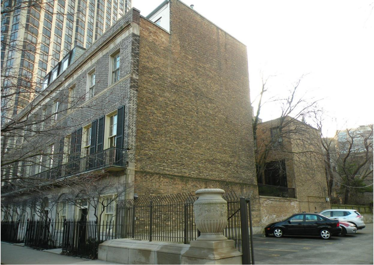
**Image 30: North elevation of number 2710 showing blank party wall for unbuilt row houses.**
