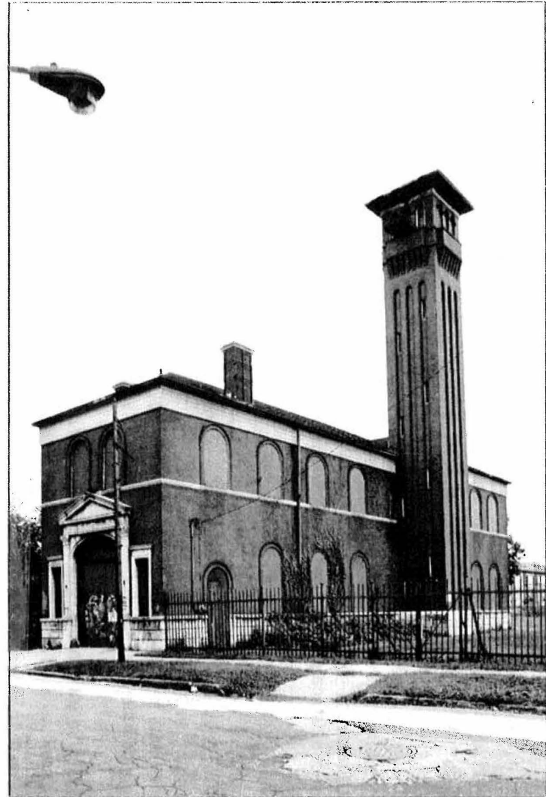
The red brick, Renaissance-inspired North Pullman fire station was constructed in the mid-1890s. The hose-drying tower is detailed by a series of tall recessed arches. (Gwen Sommers Yant, photographer)
