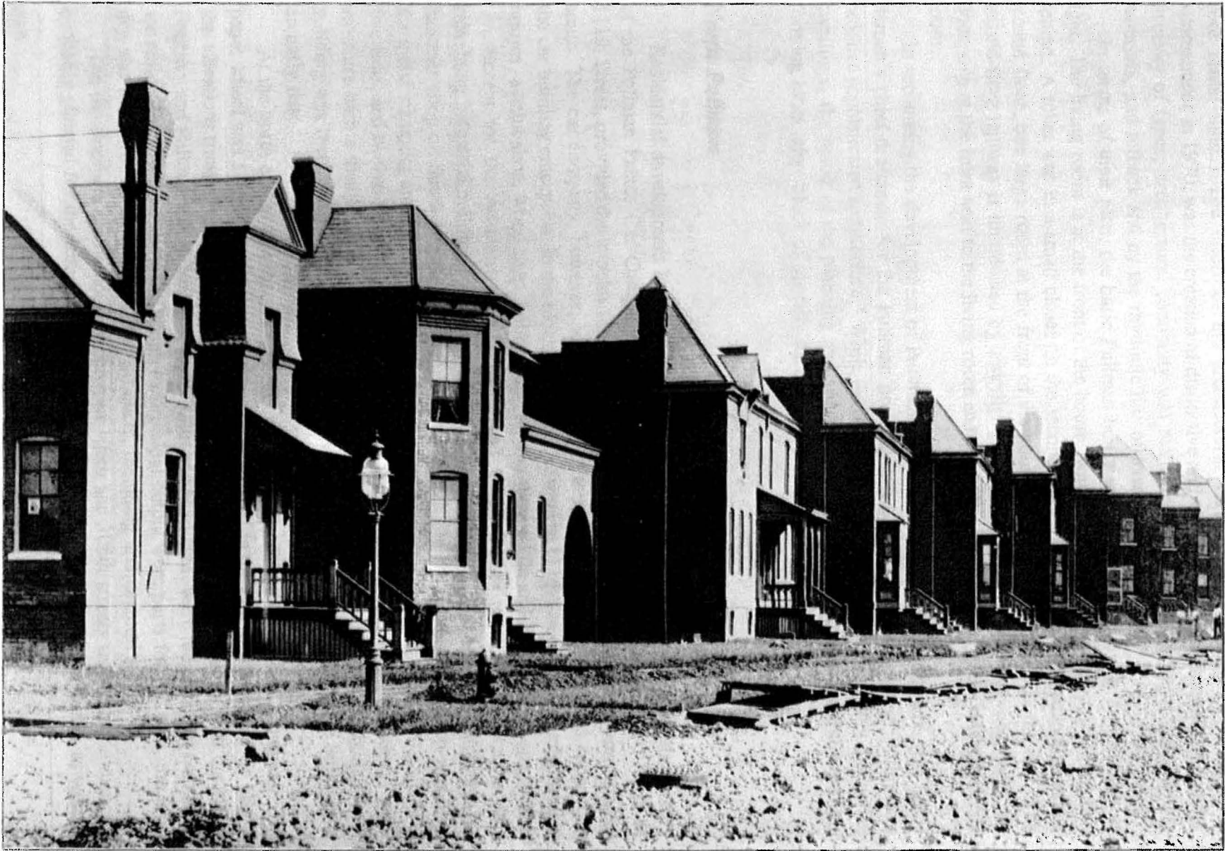
A view looking south on Cottage Grove Avenue at 107th Street, taken sometime during the late 1880s. These flat buildings, being situated on major thoroughfare, were more picturesquely detailed than comparable buildings to the west. (Photograph by J. W. Taylor; courtesy of the Pullman Research Group)
