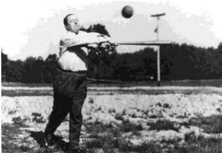
Mies van der Rohe playing baseball on the site of the Promontory Apartments.
