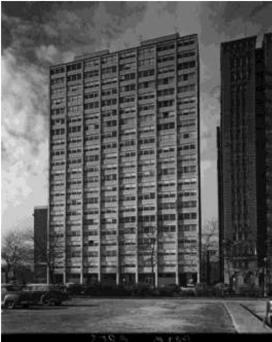
Exposed columns step back on the façade of the Promontory Apartments.
