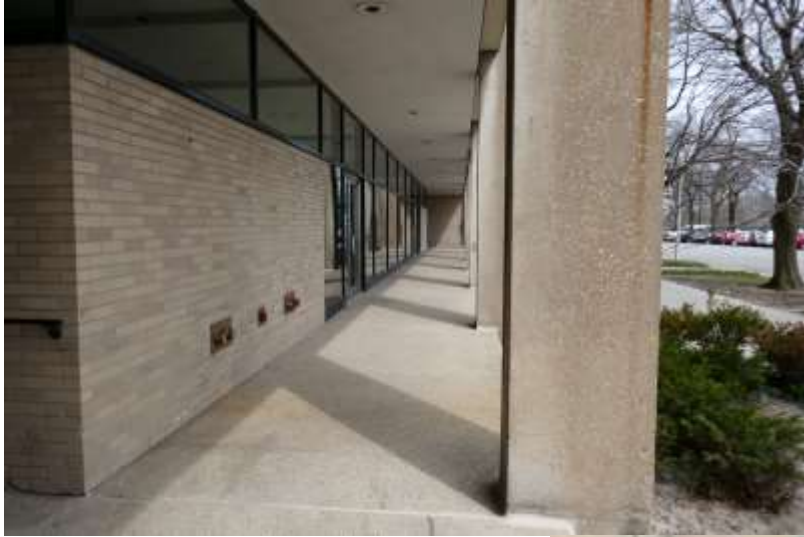
Recessed loggia at ground floor
