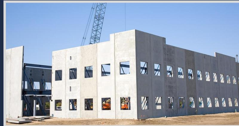
Precast concrete panel w/window openings
