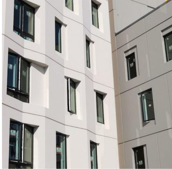
Precast concrete panels with various depths and insets
