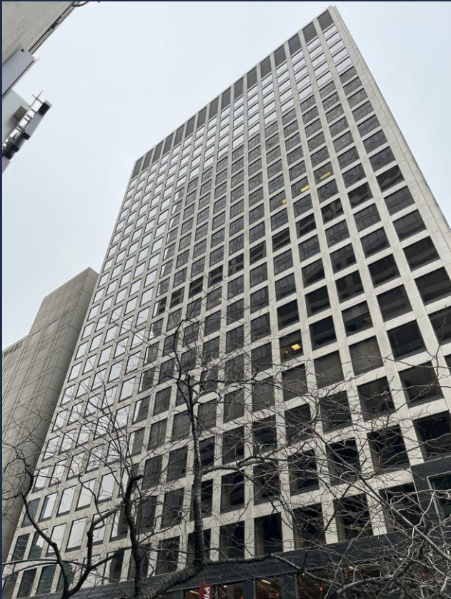
FAÇADE - MICHIGAN AVE
