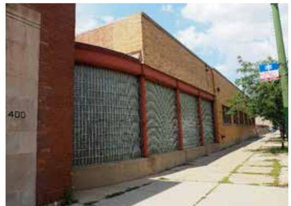
*As steel became scarce during World War II many of the buildings constructed during this time in the Kinzie Industrial Corridor used glass block in lieu of the typical steel window.*
