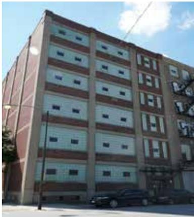
Factory: Reinforced Concrete Construction.
