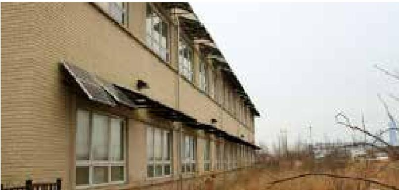
At the Chicago Center for Green Technology, solar panels serve a dual purpose, as they are used to generate electricity and are used as awnings above windows.
