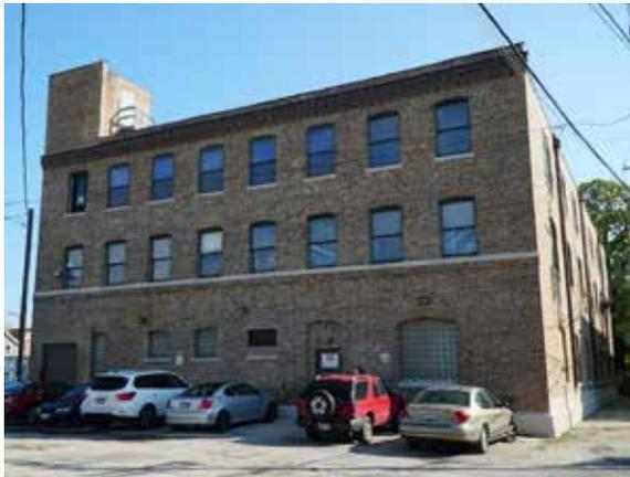
Factory: Brick Bearing Wall with Mill or Semi-Mill Construction.
