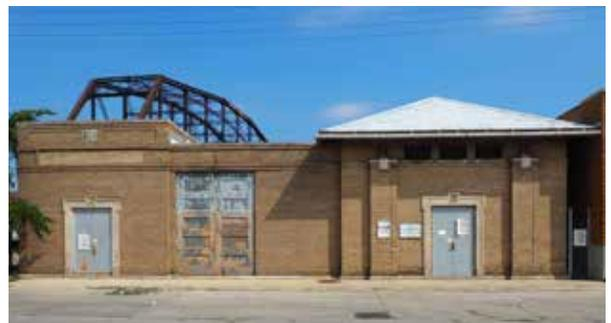
Example of brick masonry construction in the Kinzie Industrial Corridor with decorative inset terra cotta and limestone ornamentation at openings.
