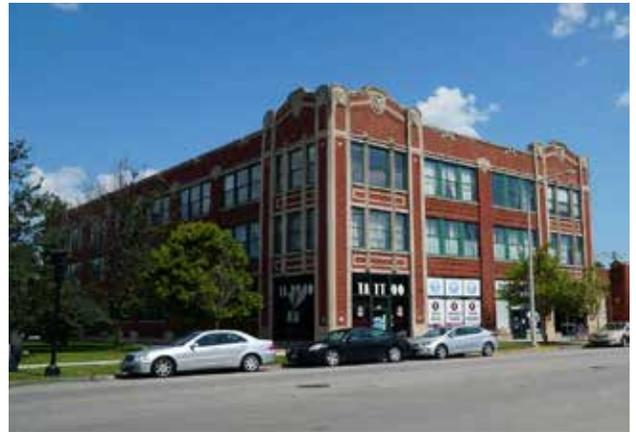
Factory: Brick Pier and Spandrel Construction.
