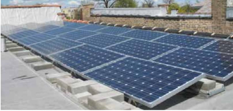
An example of a ballasted (non-penetrating) solar PV system. Here, the PV panels are not physically connected to the roof. Cinder blocks are used as ballasting means to secure the system to the roof.
