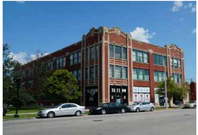
Factory: Brick Pier and Spandrel Construction.
