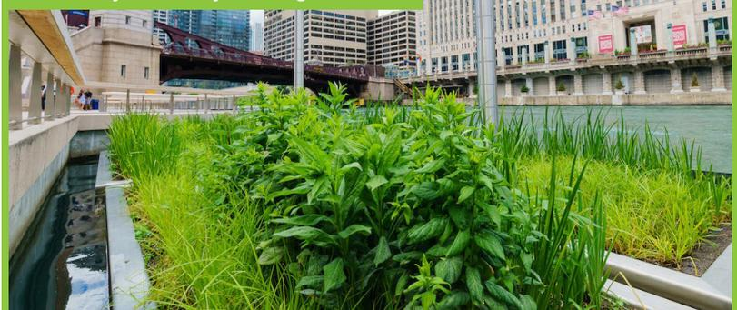
Constructed along the Jetty area of the Main Branch of the Chicago River are floating wetlands and water gardens. These floating wetlands use aquatic species to clean and improve the water, remove unwanted nutrients, and provide habitat for fish. These wetlands are constructed of a recycled plastic matrix on which aquatic and terrestrial vegetation is grown hydroponically.
