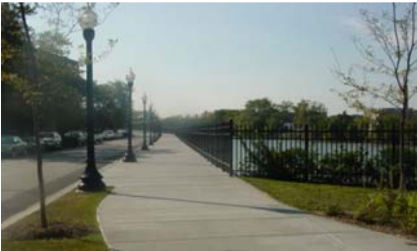
Figure 4.2 River edge lighting
