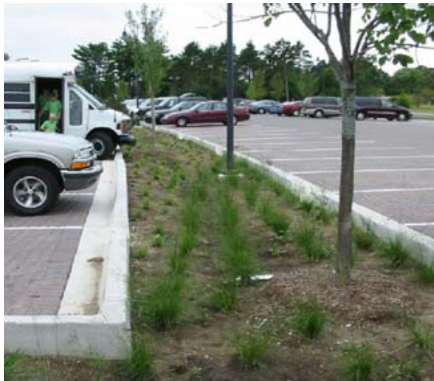
Figure 3.8 Example of Bioswale and Permeable Pavements
