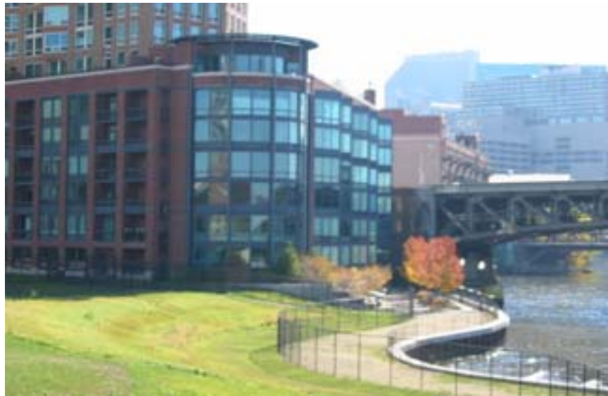
Figure 5.2 New buildings should be orientated to the river to create a safe and lively riverfront.
