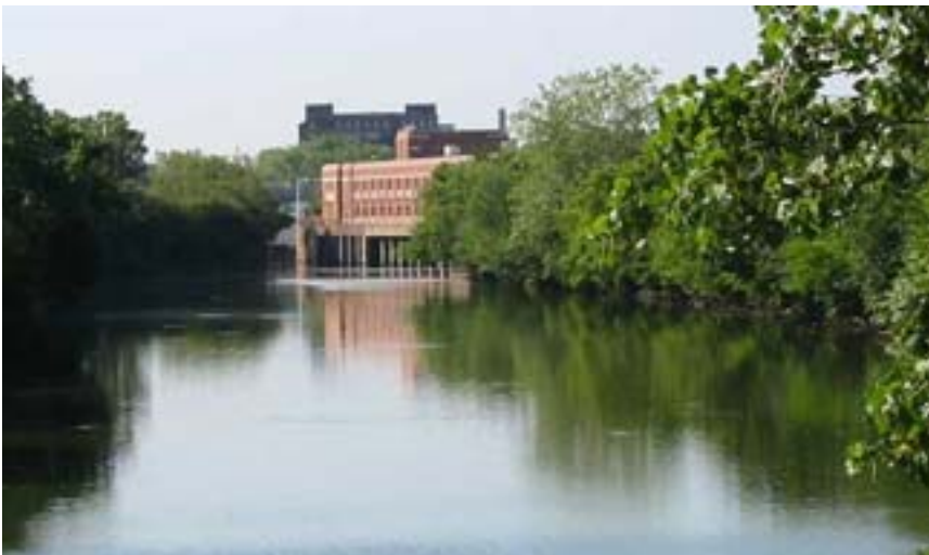
Figure 6.2 Bubbly Creek today with the Racine Avenue Pump Station in background
