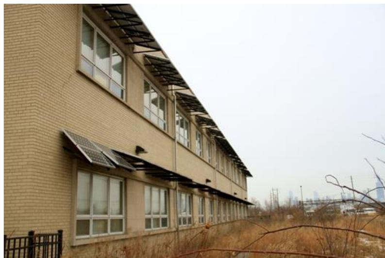
**Figure 7:** At the Chicago Center for Green Technology, solar panels serve a dual purpose, as they are used to generate electricity and are used as awnings above windows. This is an example of a non roof-mounted system. (Source: <http://news.medill.northwestern.edu>)
