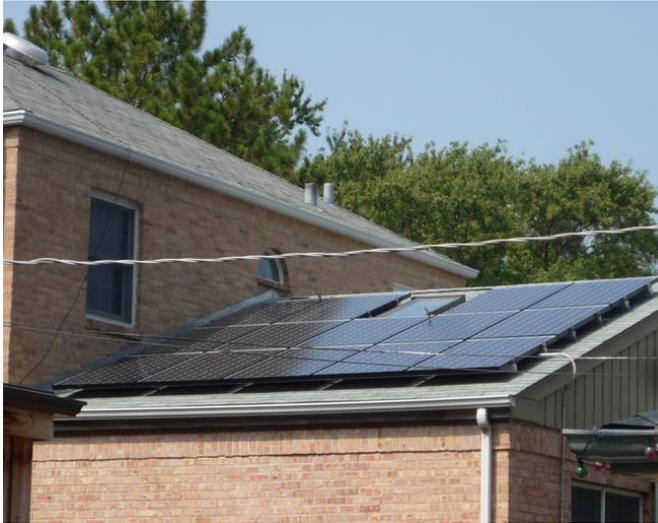
**Figure 5 (Above Left):** An example of a roof-mounted (penetrating) solar PV system
