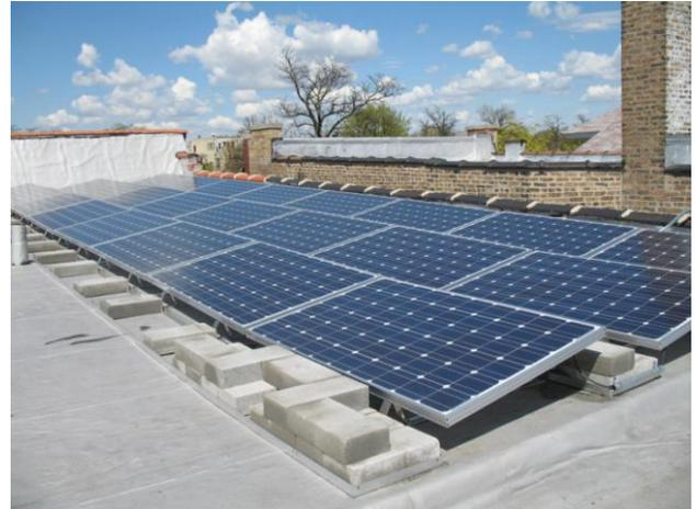
**Figure 6 (Above Right):** An example of a ballasted (non-penetrating) solar PV system. Here, the PV panels are not physically connected to the roof. Cinderblocks are used as ballasting means to secure the system to the roof. (Source: <http://www.solarserviceinc.com>)
