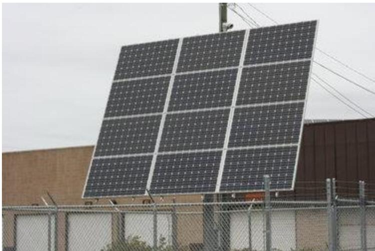
**Figure 9:** Single purpose pole-mounted solar PV system. (Source: <http://www.mlive.com>)
