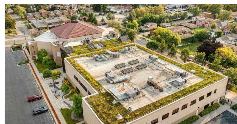
The green roof at the Trinity United Church of Christ is an example of implementing sustainable design features into buildings that can lower operating costs and improve the air quality (Source: Brook Architecture)
