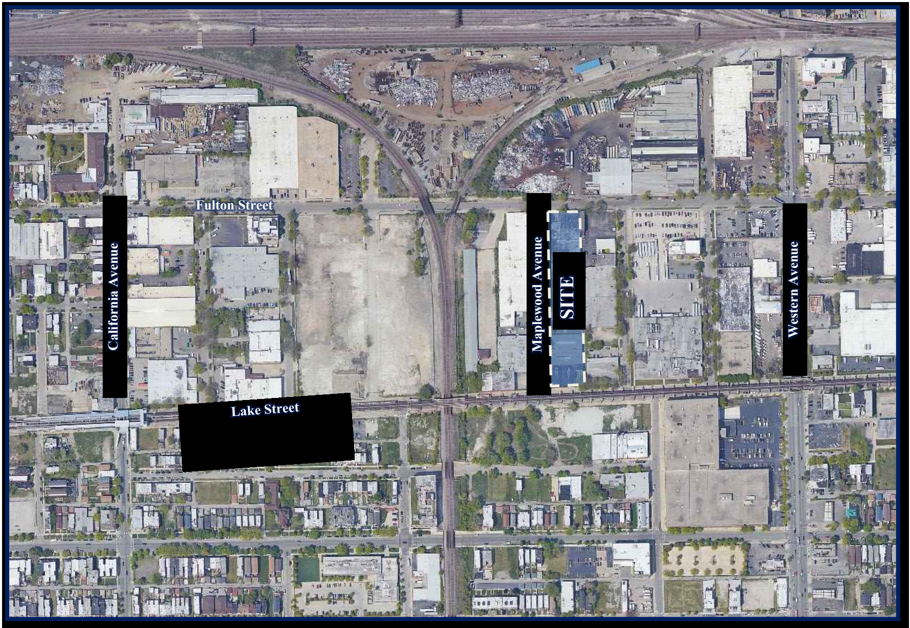
Aerial View of Site 2519 W. Fulton Street Chicago, Illinois
