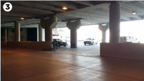
3 WEST ACCESS POINT
