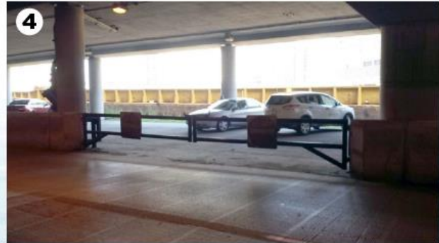
4 EAST ACCESS POINT
