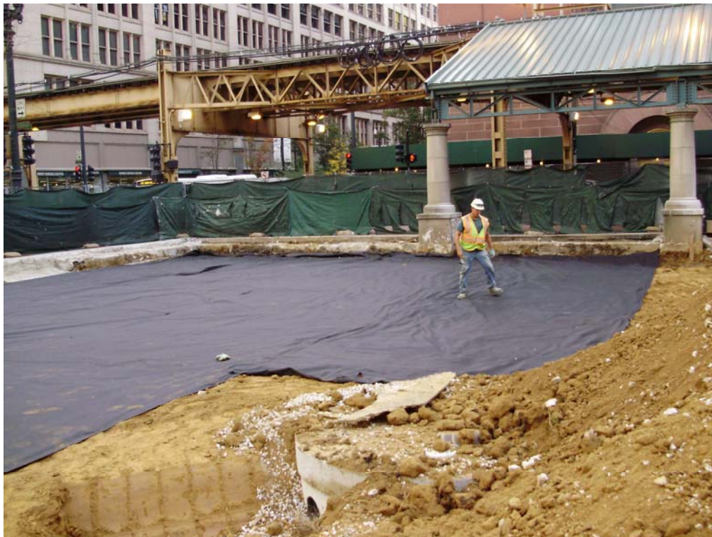
Southeast corner...PM 60-mil geotextile fabric has been installed.
