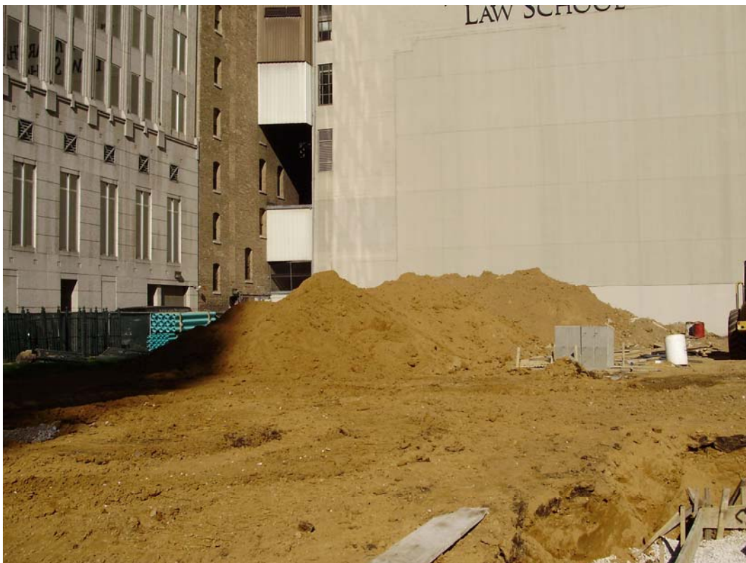
Clayey Silt soil stockpile..AM (shallow soil across site from previous re-development). This soil will be re-used within the SMZ on the west portion of the site.
