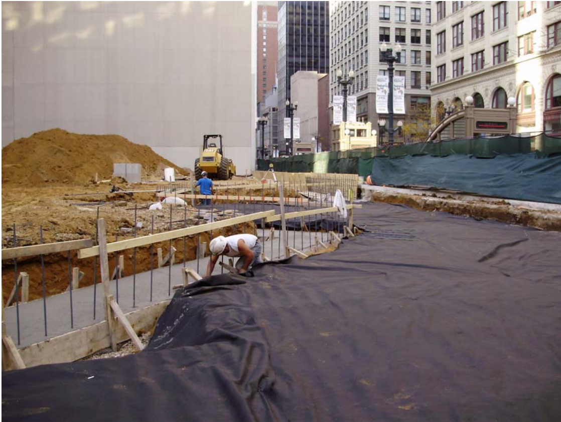
Looking northeast...PM, concrete footings have been poured over emplaced stone, geotextile installation underway.
