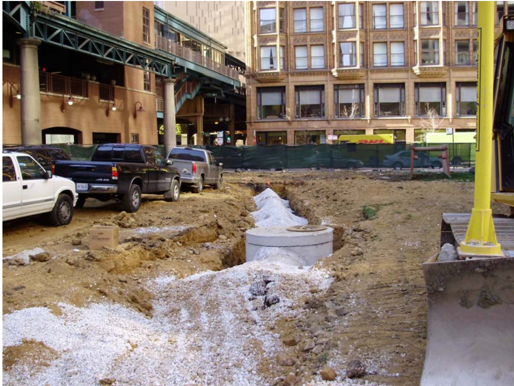
Southwest quadrant showing storm sewer re-work.
