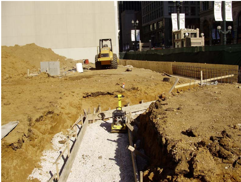
Northeast quadrant....AM w/ drainage trench and mini-compactator.
