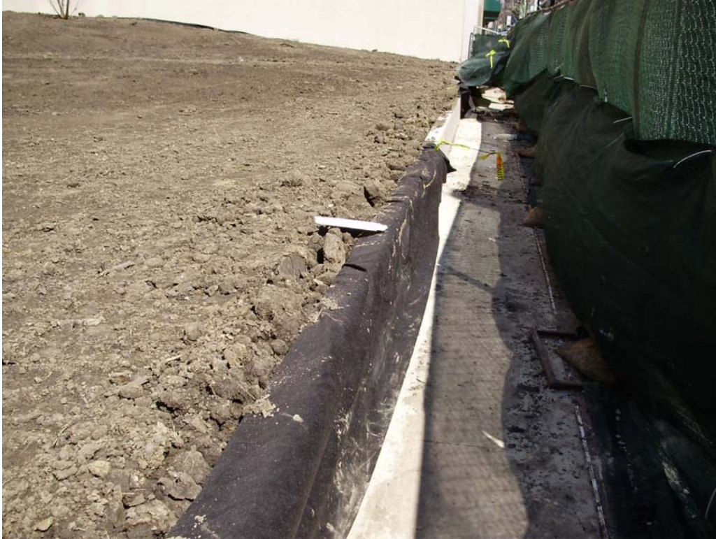
Facing north along State Street; note geotextile, 4/7/09.
