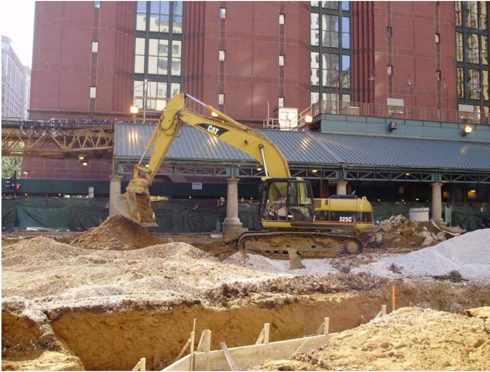
Southeast quadrant of site ....AM, recently imported stone was emplaced within Drainage basins and beneath wall foundations/footings.
