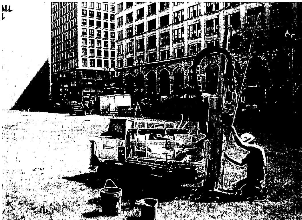
View of typical well installation activities.
