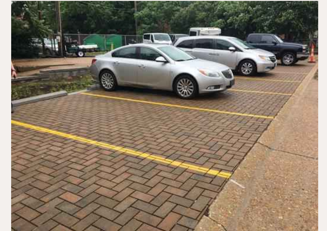
Permeable Pavement
