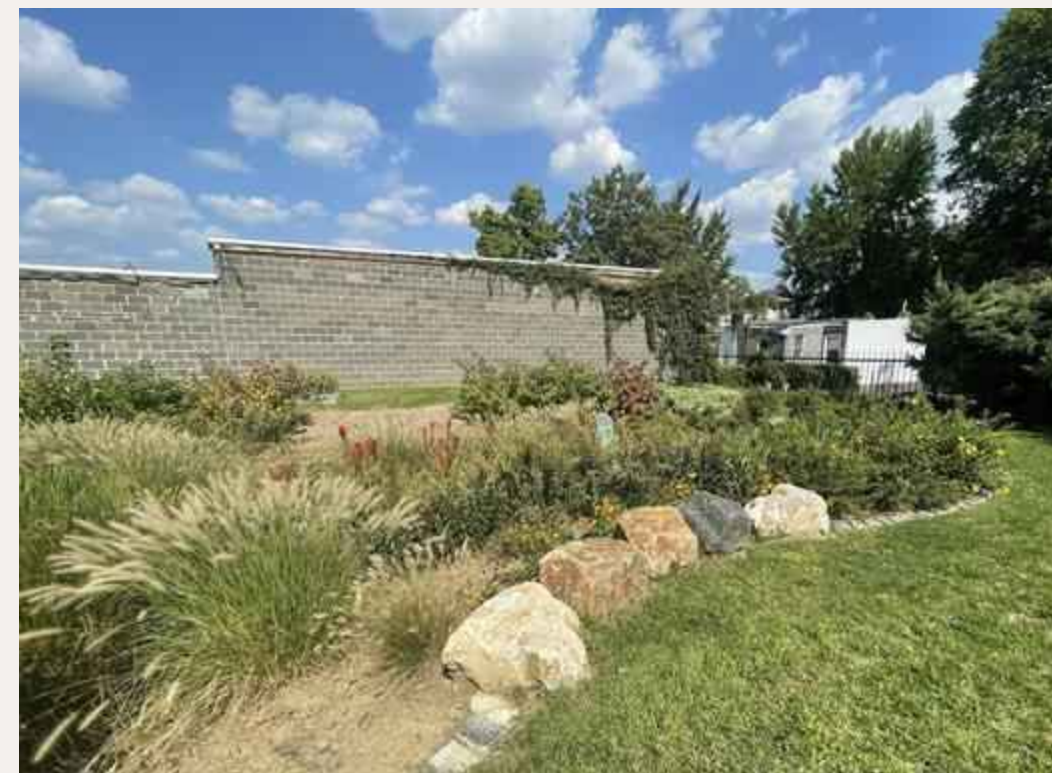
Rain Garden / Bioretention Basin
