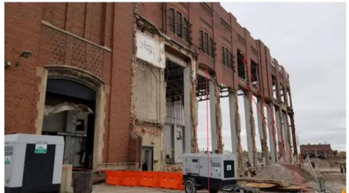
CRAWFORD POWER PLANT, SOUTH ELEVATION OF TURBINE BUILDING 5/4/20 BL01036
