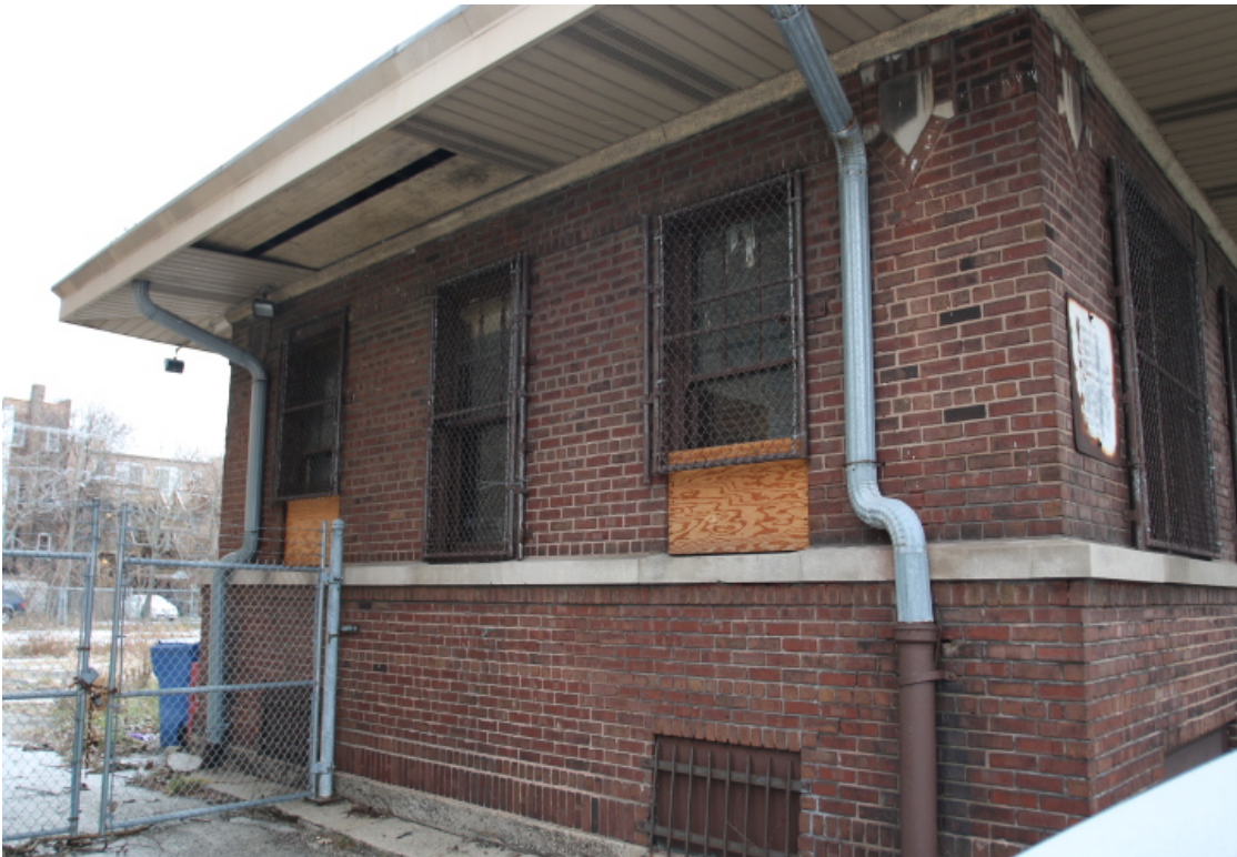
View of subject north elevation
