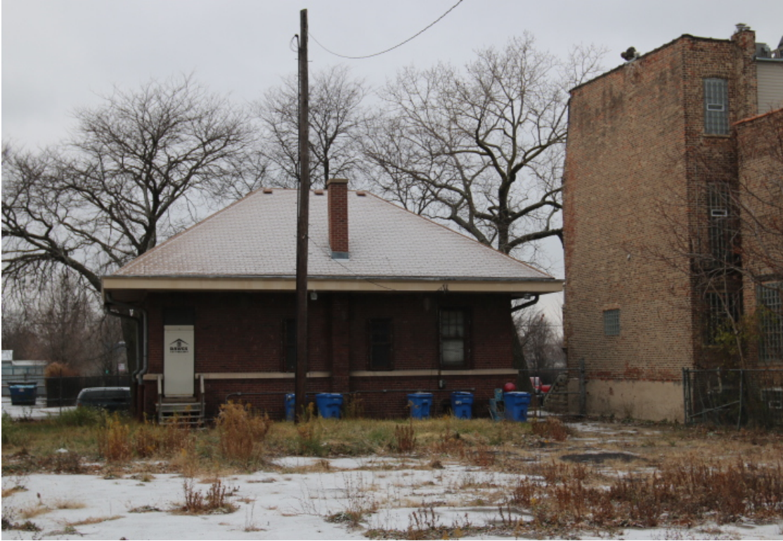
View of subject east elevation and rear lot
