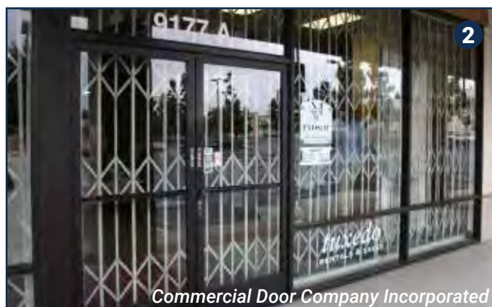
Interior mounted collapsible security gates are a discrete way to secure retail space
