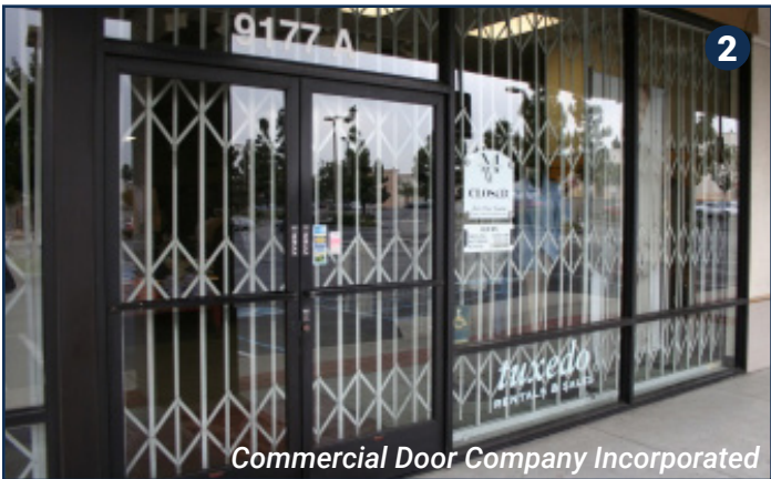
Interior mounted collapsible security gates are a discreet way to secure retail space. Commercial Door Company Incorporated
