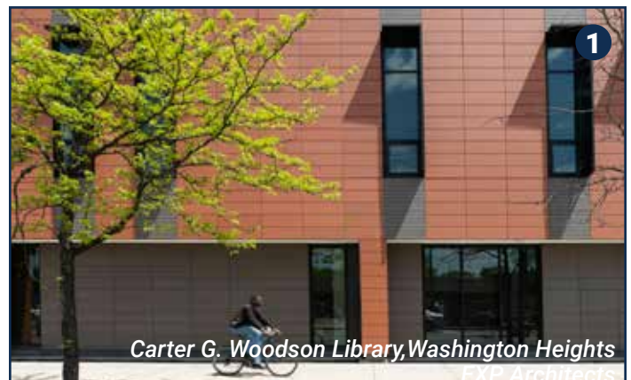
New terra cotta rainscreen curtain wall replaced a hazardous uninsulated brick facade that was falling apart
