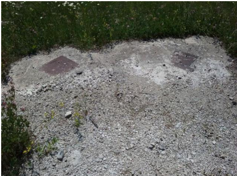
Photo 3: Closer view looking south at the metal plates. Metal plates were adhered to concrete and could not be pried up.
