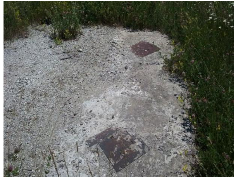
Photo 4: Closer view looking south at the metal plates. Plates did not indicate a void space beneath indicative of a UST when hit with hammer.
