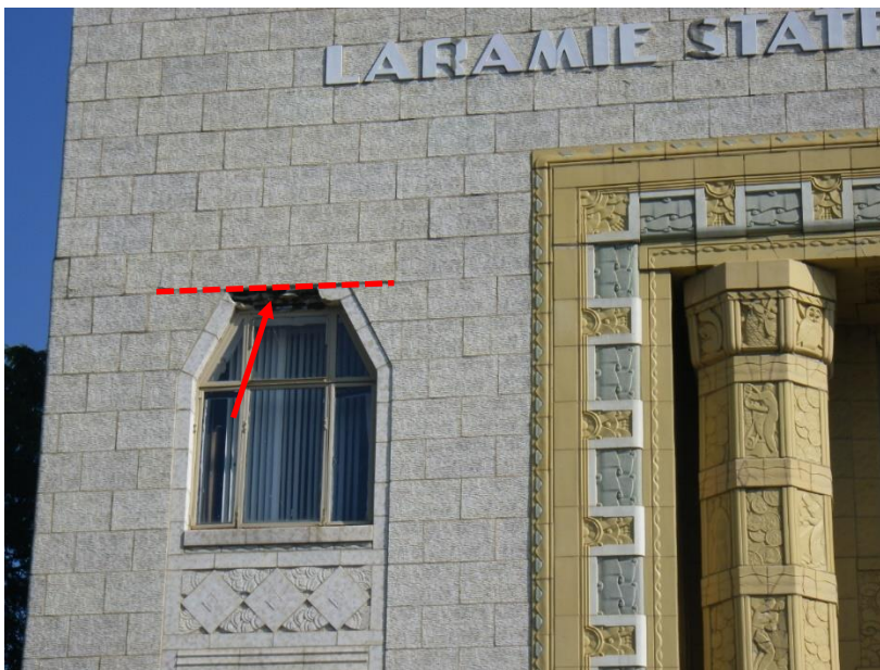
Figure 4. Missing piece of terra cotta at window head on south facade. Dashing line indicates likely shelf angle location.
