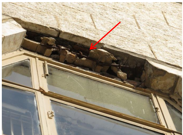
Photograph 12: Damaged and missing lintel on the south elevation.
