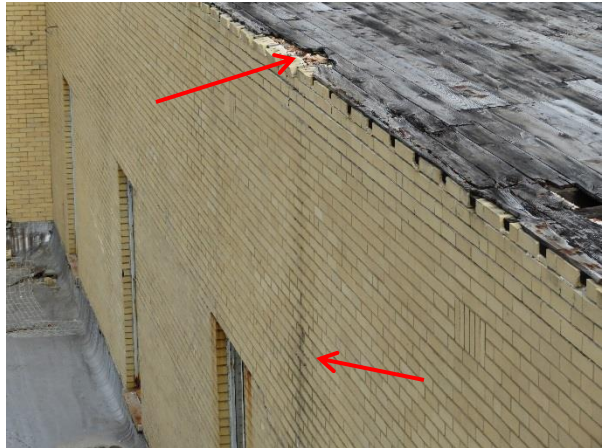
Photograph 10: Possible missing downspout and damaged edge condition at the transition from the high to the low roof.
