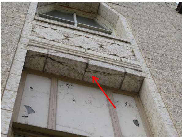
Photograph 11: Cracked decorative masonry on the eastern elevation.
