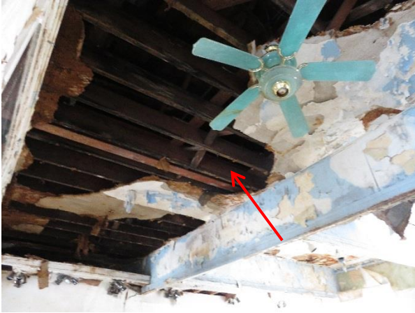
Photograph 1: Typical view of damaged finishes inside the building.
