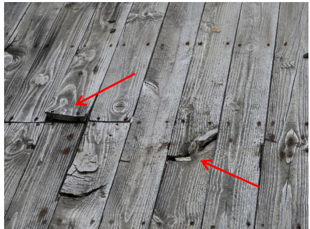
Photograph 6: Damaged roof planks at the location of missing membrane.
