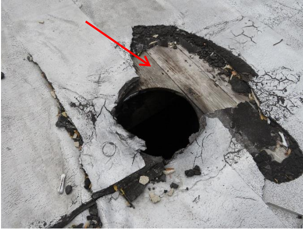
Photograph 7: Damaged membrane around a previous assumed mechanical opening.
