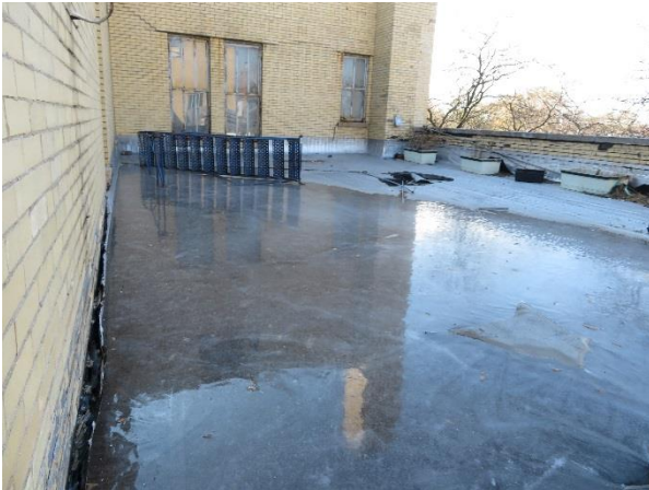
Photograph 3: Ice buildup on the low roof indicating poor drainage.
