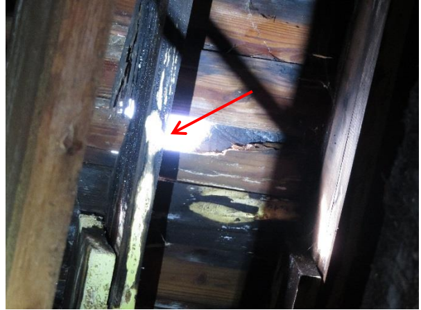
Photograph 2: Split joist near an opening in the roof.
