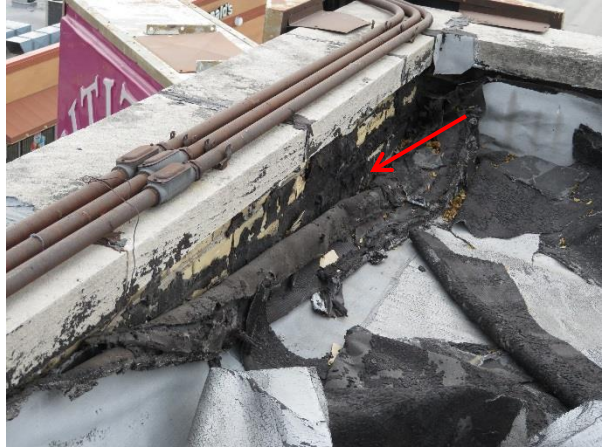
Photograph 8: Typical damaged membrane at the parapet.
