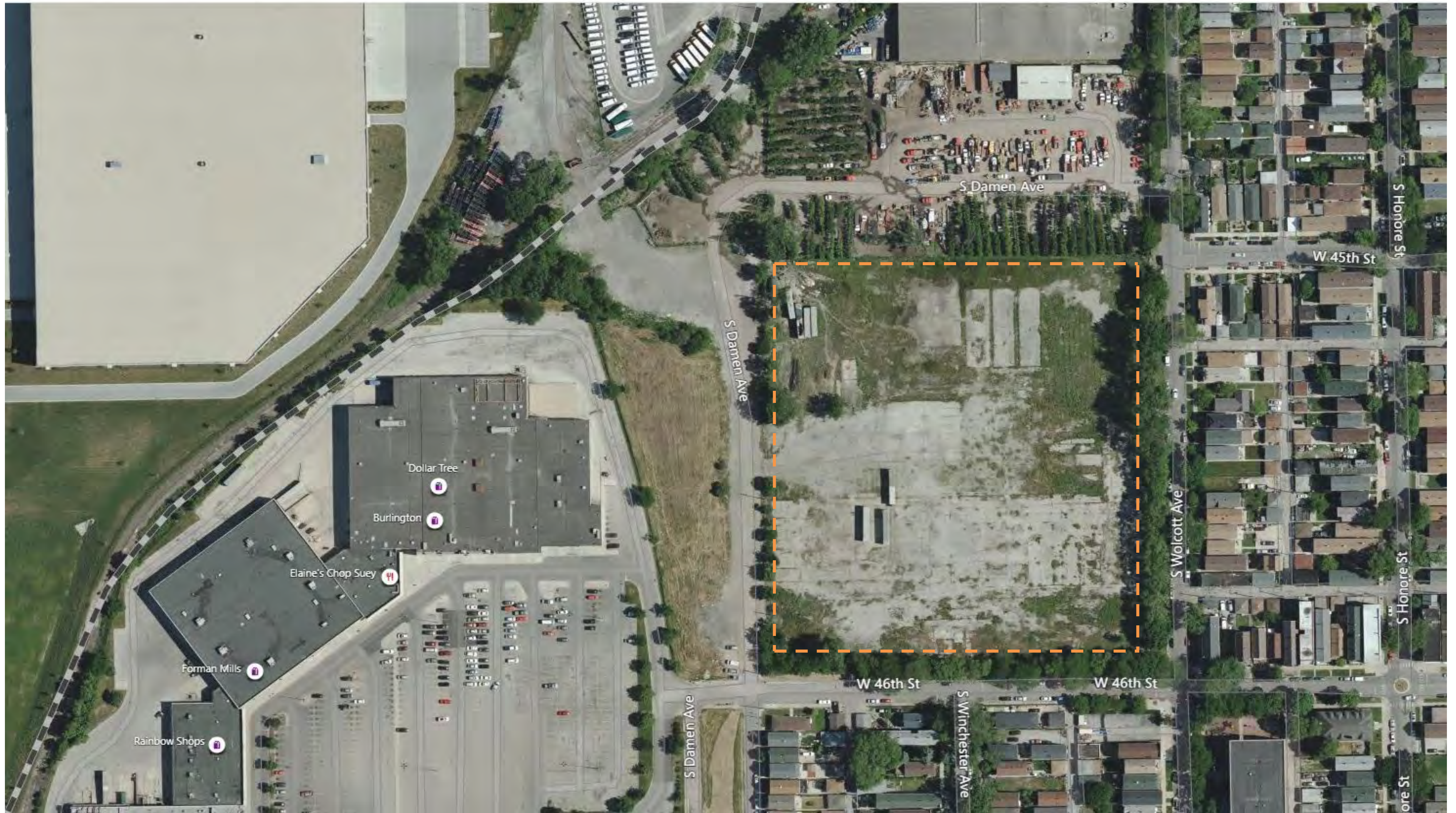
Aerial View of Site
