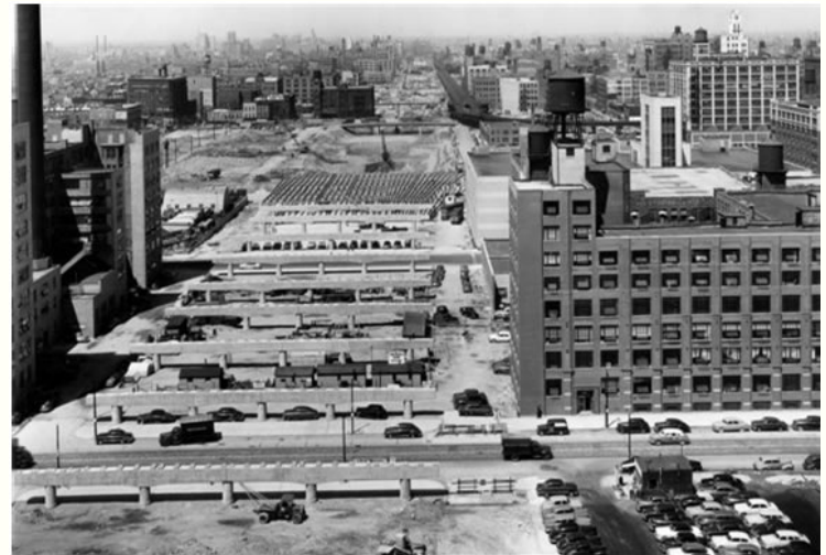
Congress Parkway construction, 1920s
