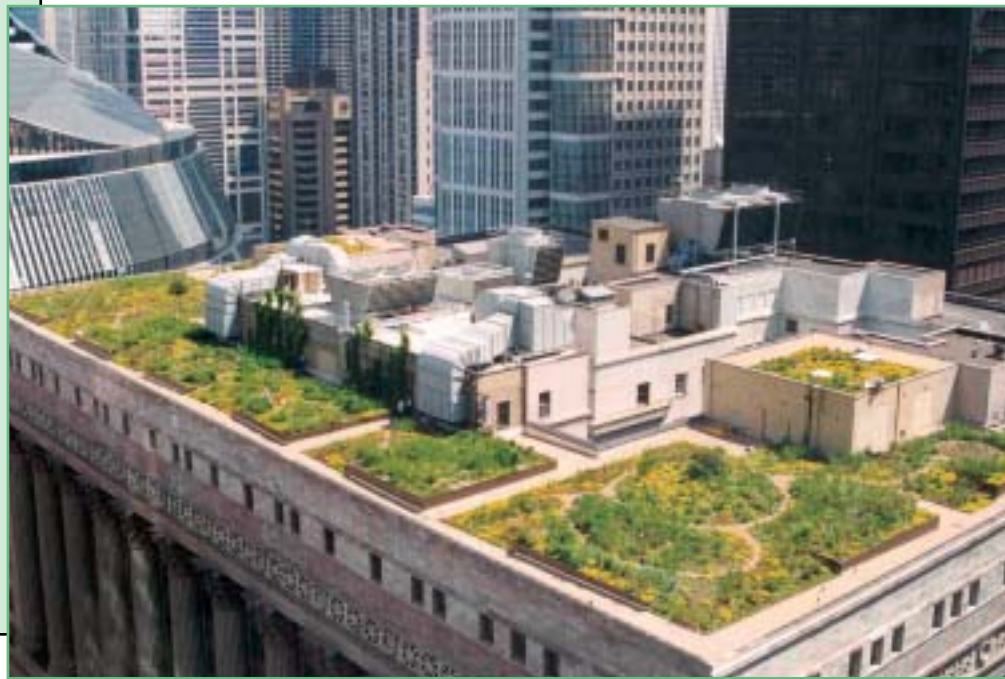
Green roof on top of Chicago's City Hall.
