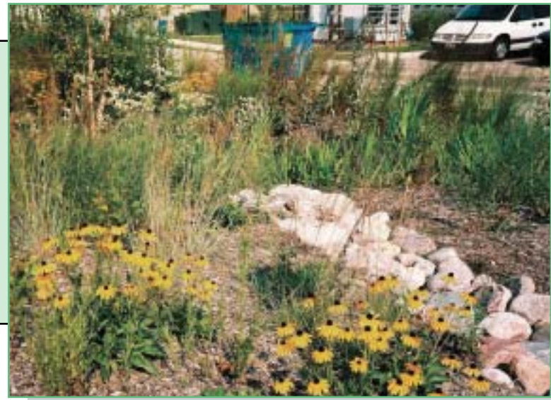
An example of a drainage swale near a parking area at the Chicago Center for Green Technology.
