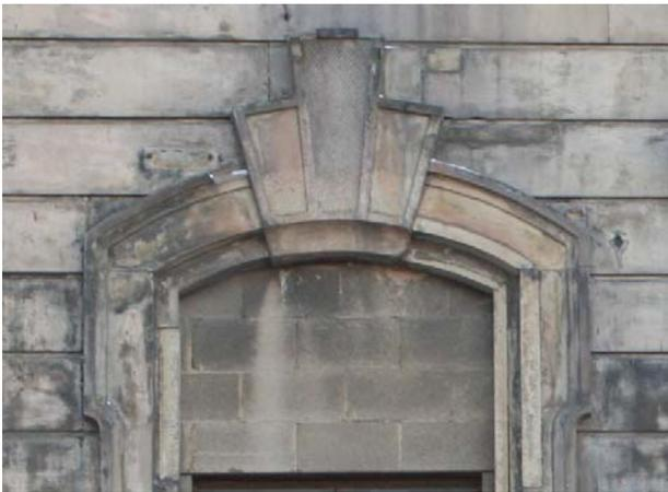
A few of the varied window surrounds in the Holden Block are shown here. Top: Round-arched paired windows with keystones from the center bay of the second floor. Left: Segmental-arched window with keystone from the side bay of the second floor. Bottom left: Segmental-arched window with crown from the side bay of the third floor. Bottom right: Flat window with rounded corners from the side bay of the fourth floor.
