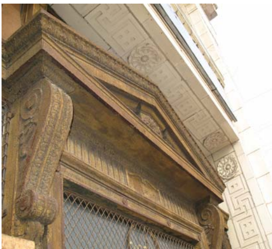
The building's main entrance is finely detailed with Classical ornament, including a bracket-supported triangular pediment.
