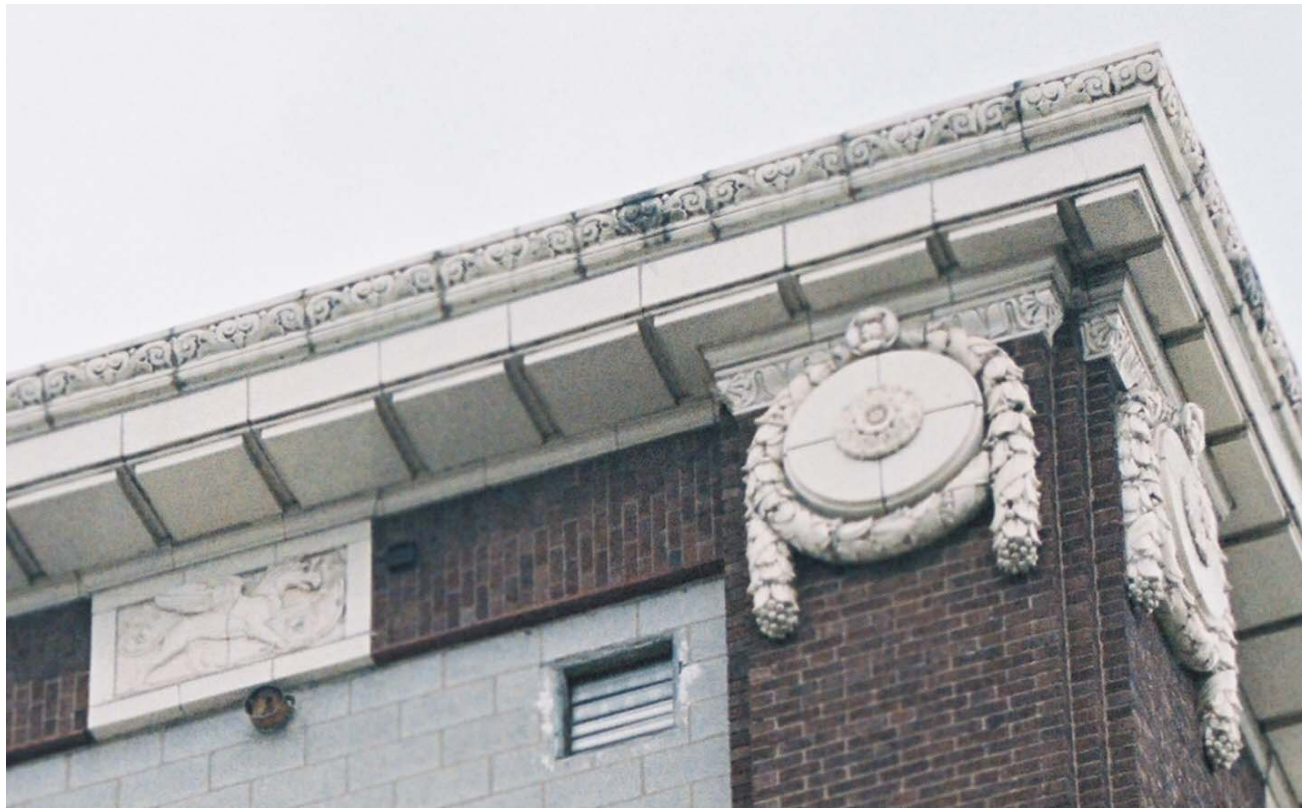
A detail of the building's cornice and roofline ornament.
