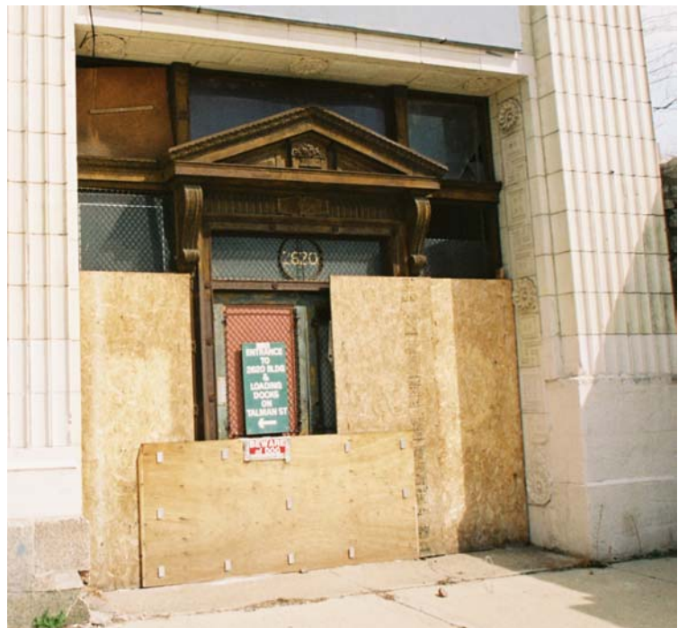
The building's main entrance is finely detailed with Classical ornament, including a bracket-supported triangular pediment.
