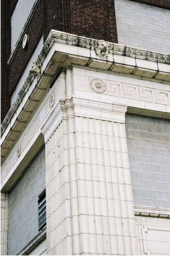
The exterior of the Lindemann & Hoverson Company Showroom and Warehouse Building features a handsome terra-cotta base with fluted pilasters, Greek-key designs, rosettes, and lion-head ornament. The capitals of the brick piers have central rosettes and draping garlands, while griffin-decorated panels are located under the projecting cornice.
