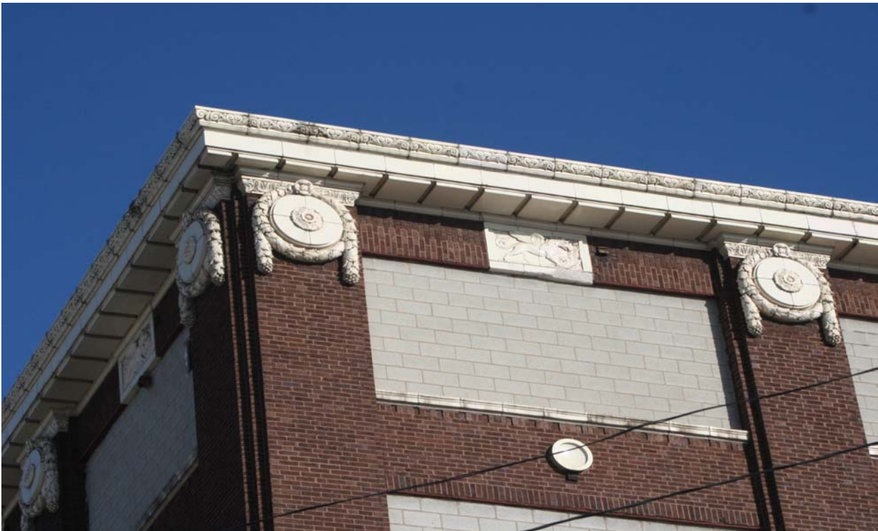
The exterior of the Lindemann & Hoverson Company Showroom and Warehouse Building features a handsome terra-cotta base with fluted pilasters, Greek-key designs, rosettes, and lion-head ornament. The capitals of the brick piers have central rosettes and draping garlands, while griffin-decorated panels are located under the projecting cornice.
