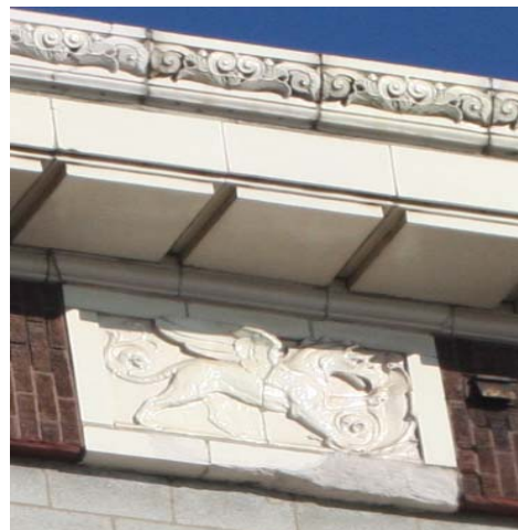
A detail of one of the griffin-ornamented panels under the foliate-detailed cornice.
