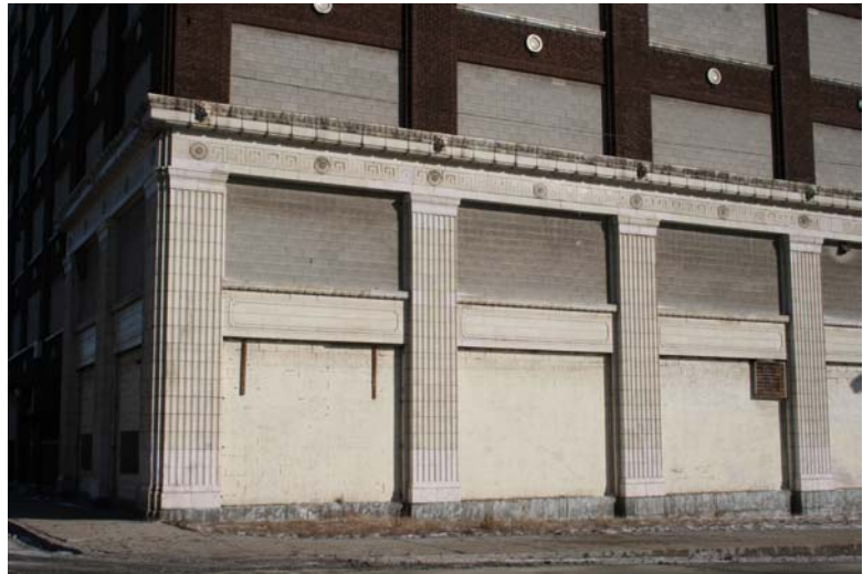
The Lindemann & Hoverson Company Showroom and Warehouse Building stretches along N. Talman Ave. with its main entrance facing Washington Blvd. And its eastern elevation abutting the Chicago & North Western Railway viaduct. Built in 1924, the flat-slab, reinforced-concrete loft structure was designed to house a first-floor showroom facing Washington Blvd., plus upper-floor storage.
