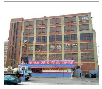
The Spiegel Administration Building's street (south) elevation features continuous spandrel panels and recessed vertical piers of red face brick that frame large rectangular window openings. The building's concrete structural system is clearly expressed on the east and north elevations, which house original multi-light steel sash windows.
