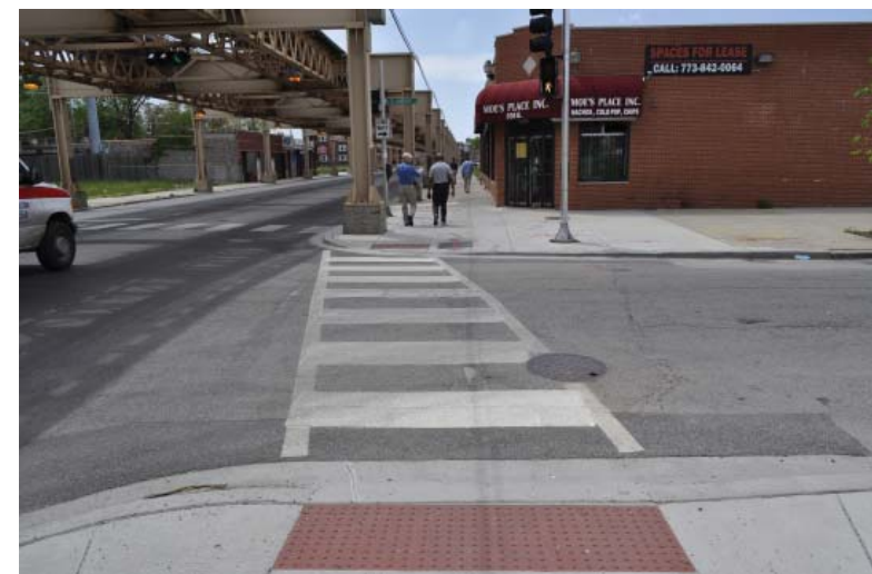
CROSSING THE STREET View looking West. Street crossings are marked with crosswalks but align to obstructions in the walkway such as the L column above. The width of the crossing can be narrowed to provide a level of comfort for pedestrians to cross the street. Due to the small turning radii of the streets, the crossings are very close to the turning movement of the intersections, creating an unsafe environment.
