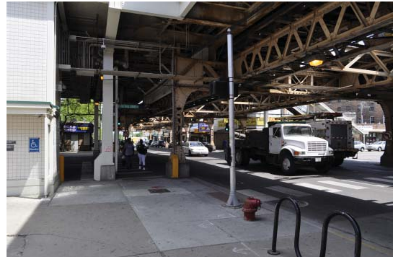
PEDESTRIAN ACCESSIBILITY Though the sidewalk is wider in this area, the amount of miscellaneous furniture, columns and sign posts block pedestrians and limit vehicular views.
