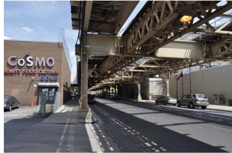
BUILDING PROXIMITY Due to the scale of the buildings and proximity to the L structures, pedestrians feel confined along this section of the corridor. (Note the security fence on top of the building.)
