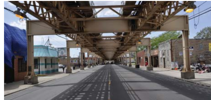
VIEW WEST TOWARD THE KING DRIVE STATION. note the wide travel lanes, lack of street trees and narrow sidewalks. The L structure consumes a good portion of the sidewalk making it difficult for pedestrians to walk the corridor.
