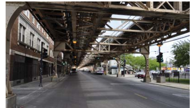
VIEW WEST ON 63RD STREET AT THE KING DRIVE STATION
