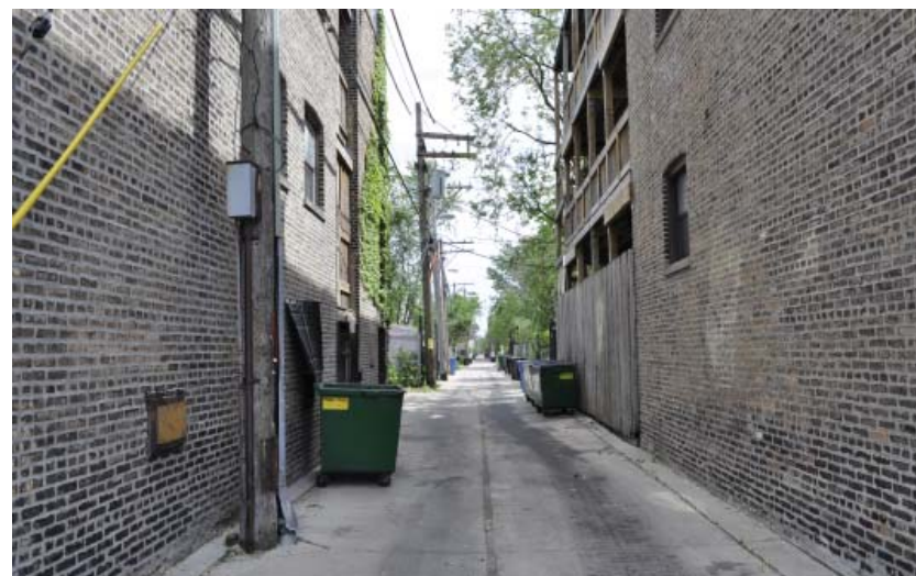
TYPICAL ALLEY VIEW The alley not only serves as a transition point between land uses, but it helps to enhance the overall street connectivity as well as provide a screened space for back of house uses.
