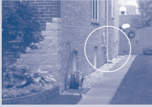
This is an example of a site where the downspout should not be disconnected. Water will make the path icy in winter.
