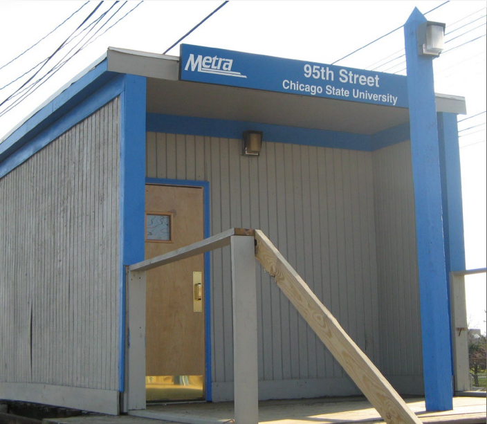
Existing Stair Headhouse
