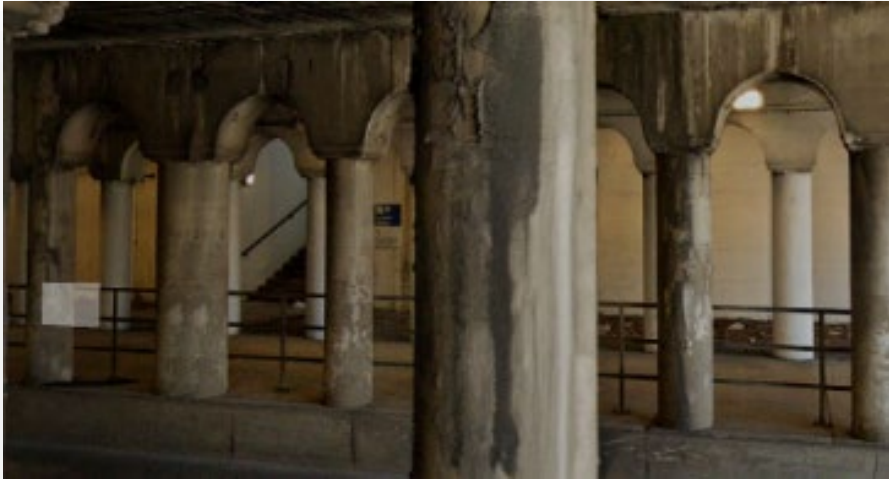
Existing Entrance, Street View
